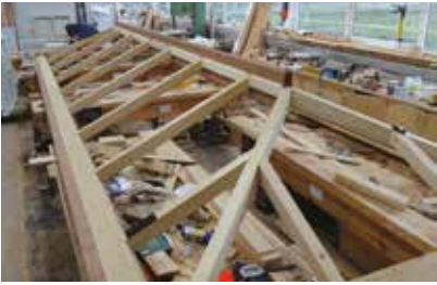
A roof lantern light under construction
